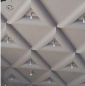
Figure 7.- Detail of the ceiling
