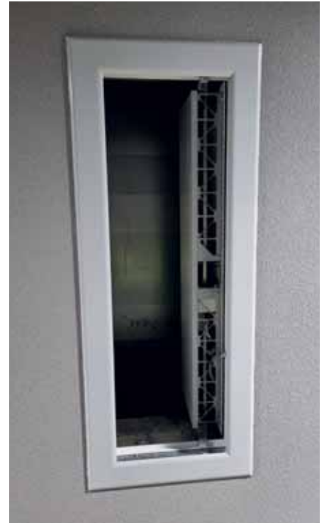
Brandwerende rookklep, conform EN12101-8 multi compartiment: in geopende toestand, op de brandverdieping tijdens brand.
