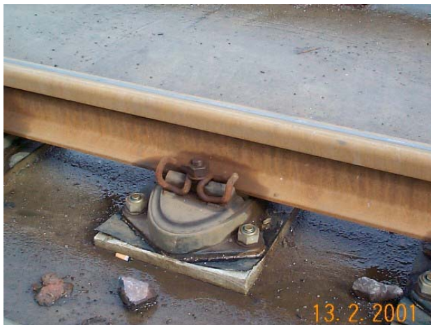
Figure 6: Example of a rail mounted on a rubber rail pad
